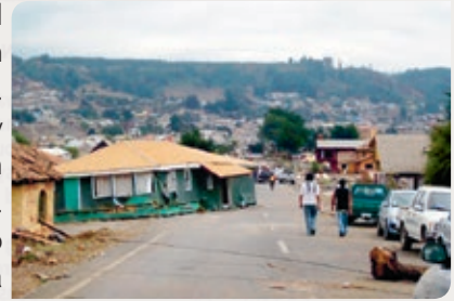
Pelluhue after the earthquake.
